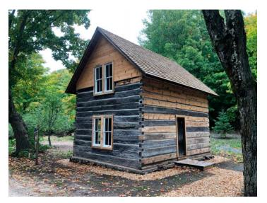
the timbers and carefully inspected each timber. All of the red pine timbers were found to be in good condition and some yellow birch timbers could be saved and restored. Unfortunately, ten of the original birch timbers were badly deteriorated and required replacement.
